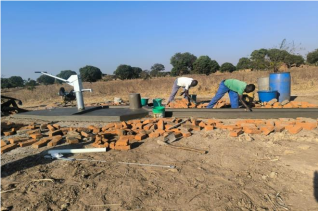
The borehole in Matekwe village during Apron construction
