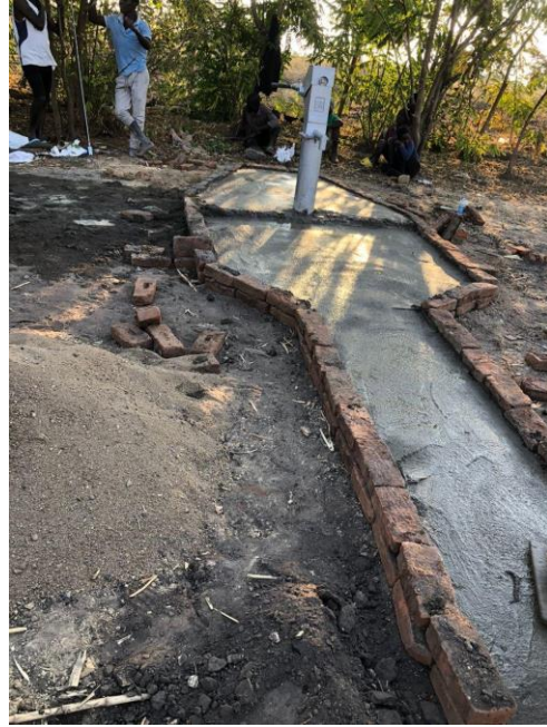
Left - New borehole in Mfungulu village before commissioning, Right- Construction of Aprons for the newly constructed borehole in Chilemba village during the month.
