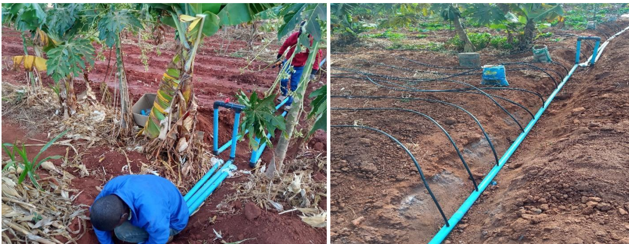
Installation of drip system on OCA agroecology farm
