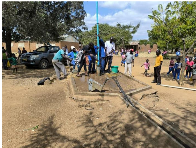
Water point repair session at Mkuyu Primary School during the month
