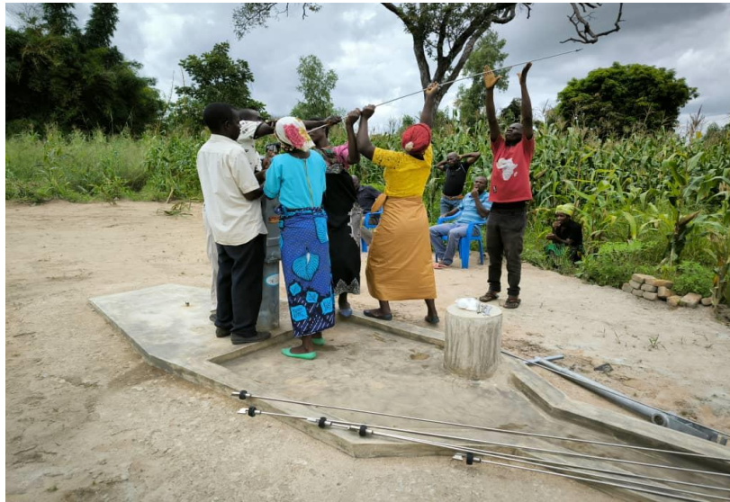
Water well repairs in progress with Community Participation
