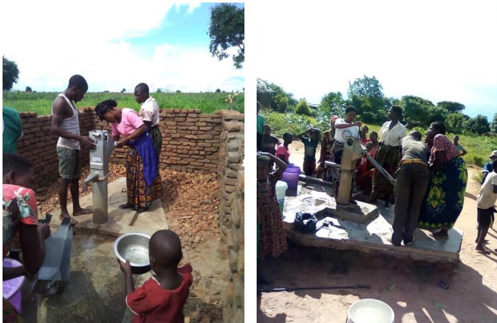
Afridev pump Area Mechanics performing borehole repairs during the month
