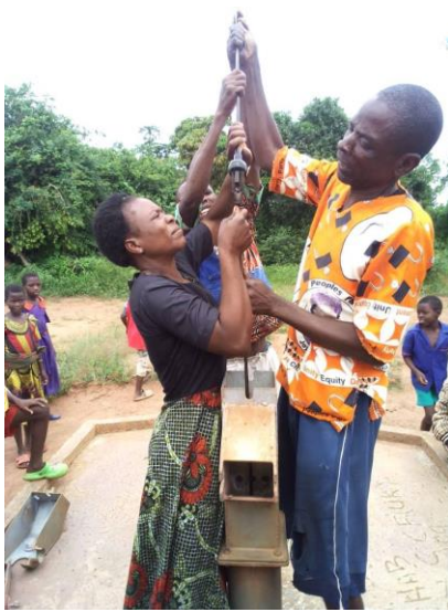
Female Afridev pump Area Mechanics performing borehole repairs during the month
