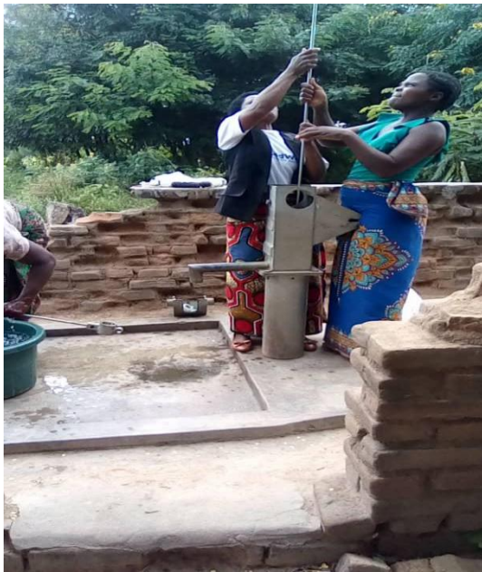
Left - Area Mechanic conducting preventive maintenance of Afridev pump in Shawa village during the month, Right- Preventive maintenance in Ntanda village
