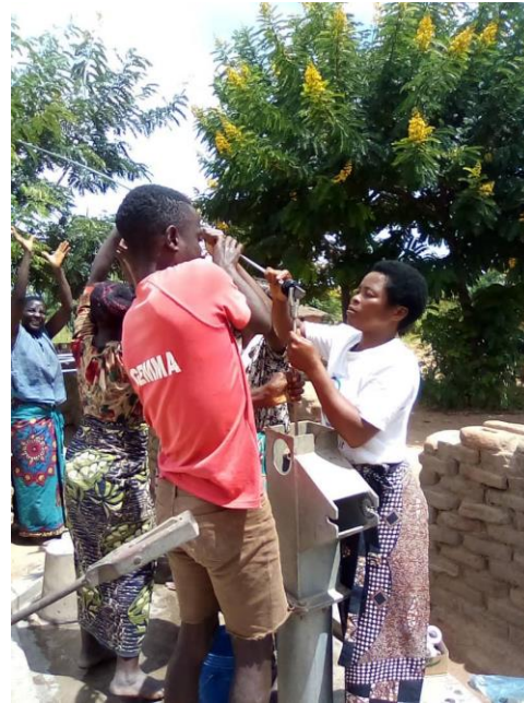
Left - Area Mechanic conducting preventive maintenance of Afridev pump in Shawa village during the month, Right- Preventive maintenance in Ntanda village
