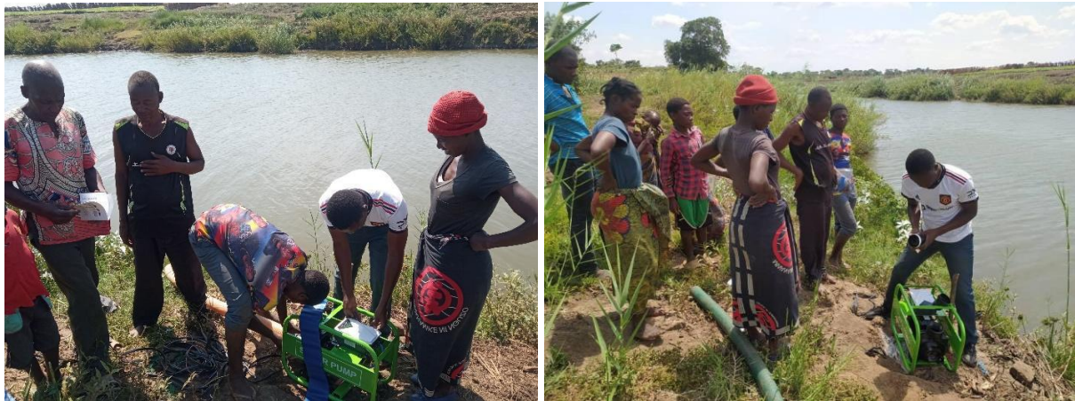
Installation of solar pump at Kambalani irrigation club
