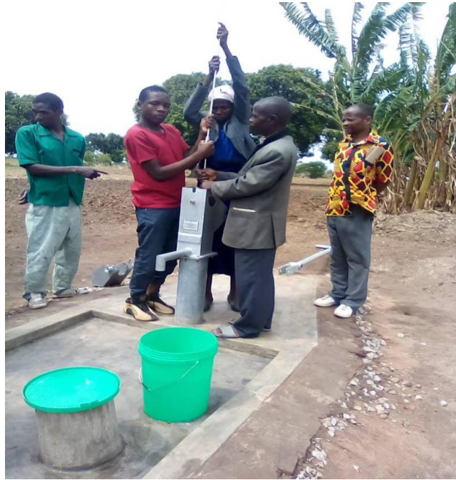
Borehole repair during the month
