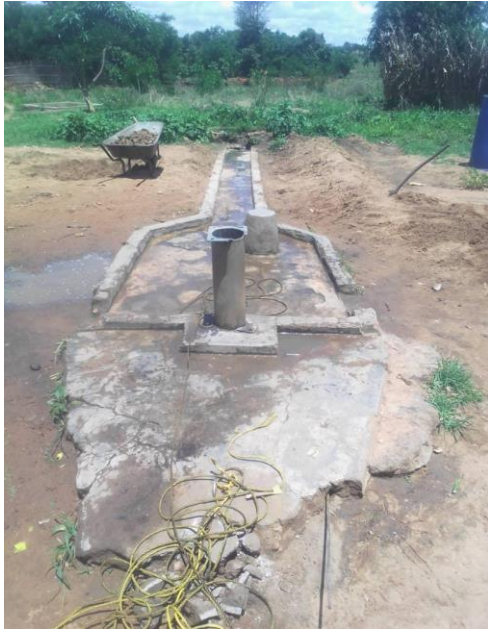
Left: Damaged apron of a borehole, Right: Rehabilitated borehole apron with support from OCA
