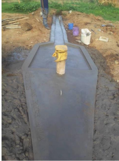
Left: Damaged apron of a borehole, Right: Rehabilitated borehole apron with support from OCA
