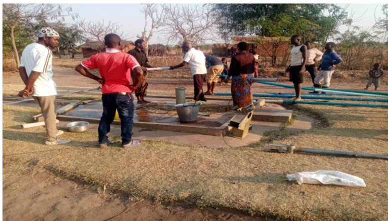
Area Mechanic repairing a pump during the month
