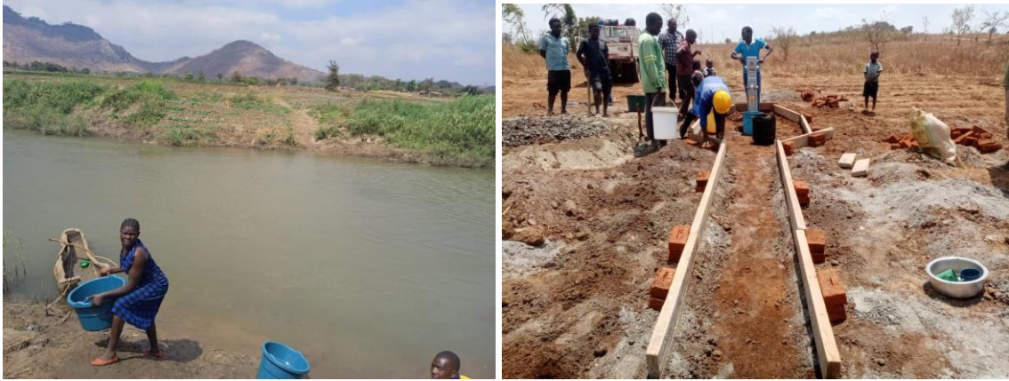
Left -A woman collecting water from the river in Chika village before OCA intervention Right - A dawn of hope; a newly constructed water point in Chika village during the construction of the Apron
