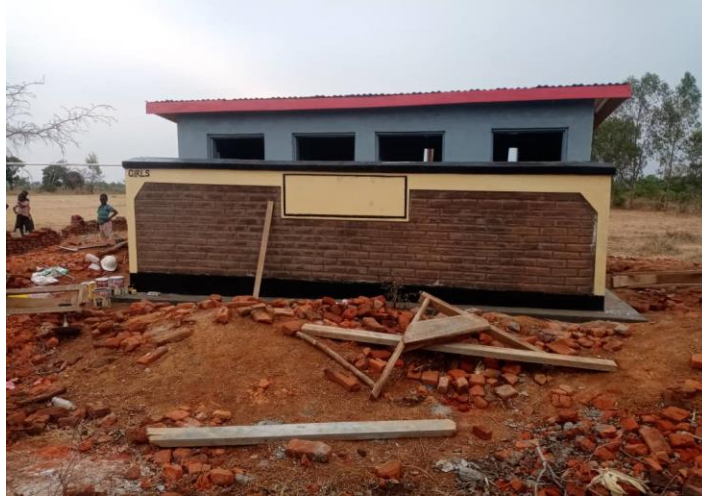
Construction of girl's latrine at Kalikulu Primary School before handover
