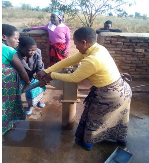
Area Mechanic repairing a pump in Mphongole village
