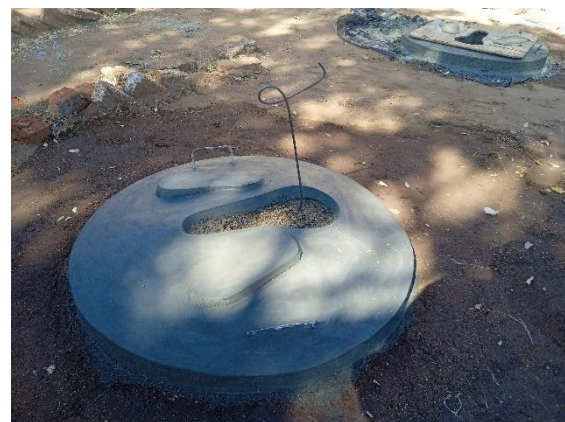
Left above – Early stages in the construction of a dorm-shaped pit latrine slab, Right above – Completed dorm-shaped pit latrine during the sanitation entrepreneurs' training
