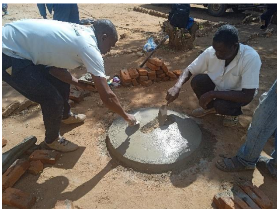
Left above – Early stages in the construction of a dorm-shaped pit latrine slab, Right above – Completed dorm-shaped pit latrine during the sanitation entrepreneurs' training
