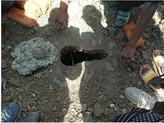
Left above – Finalized corbelled latrine substructure construction pending construction of the superstructure,
