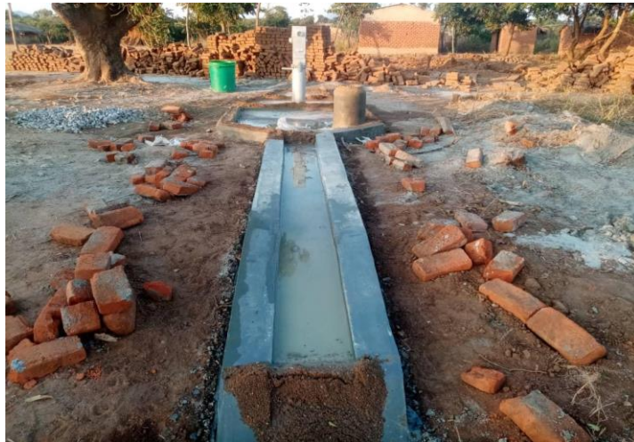
Newly drilled well at Nambola School before handover
