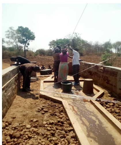
Image showing borehole repair in progress.
