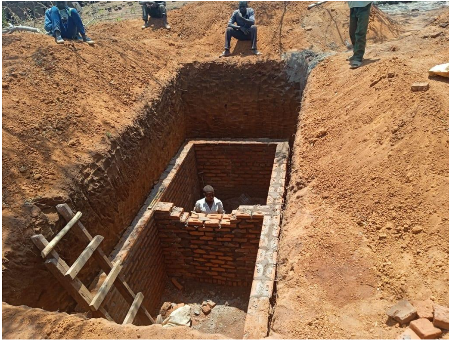
A pit for the first latrine at Kapini primary school
