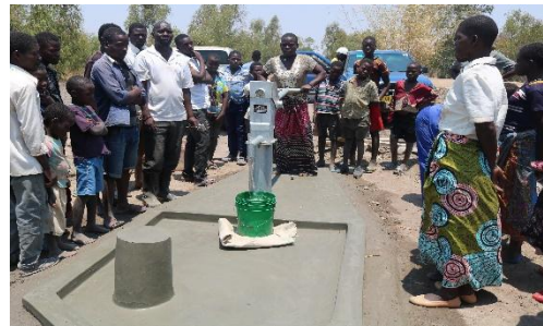
New Borehole drilled by OCA in Zindo
