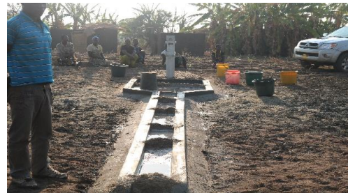
Newly drilled borehole before opening
