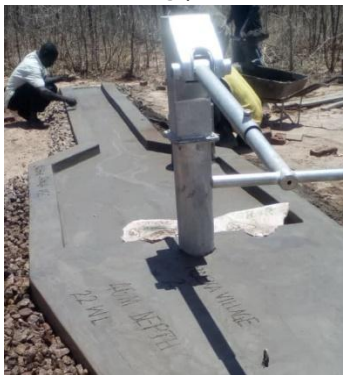
Civil works in progress on the new borehole
