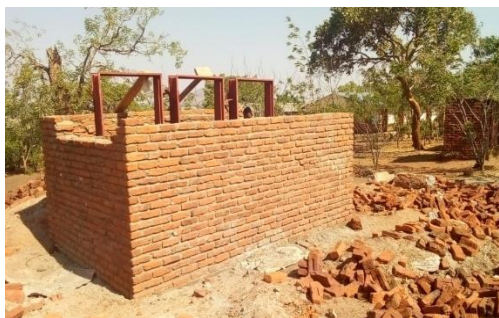
Figure 7: Construction at superstructure level
