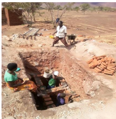
Figure 6: Latrine at a substructure phase
