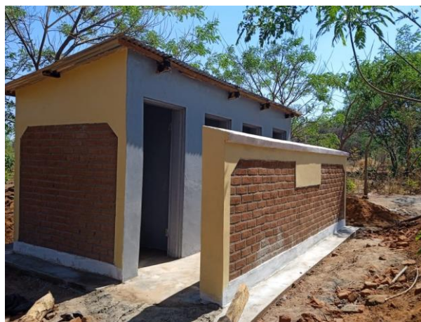
Progress of latrine construction at Kapini school
