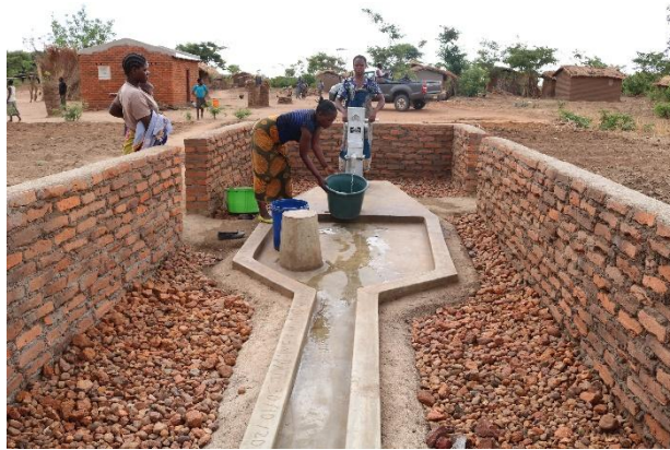
Newly drilled borehole in Mzimuwakana village during fence construction
