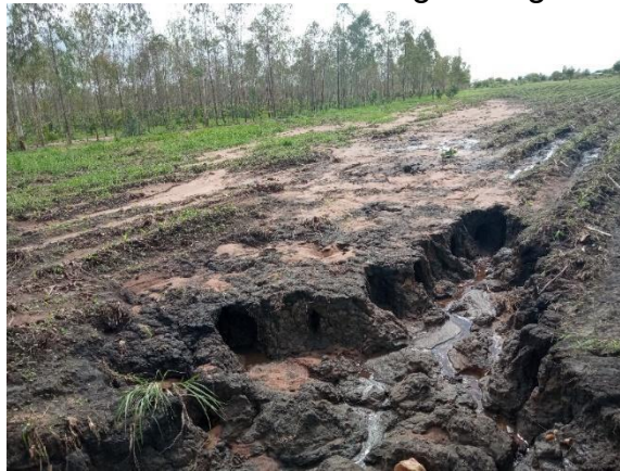
Part of OCA farm affected heavily with high speed running water
