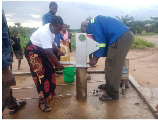
Borehole repair session with Area Mechanics in Chimbalu village
