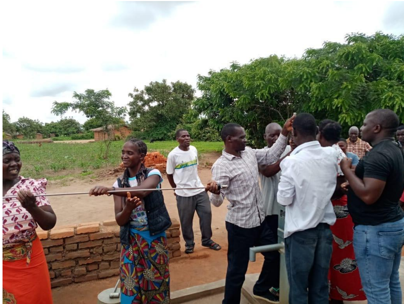
Practical training on water well repairs
