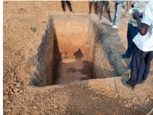
Left - Current status of pit latrines at Madzo primary school, Right - A pit for new latrines being constructed by OCA at Madzo primary school
