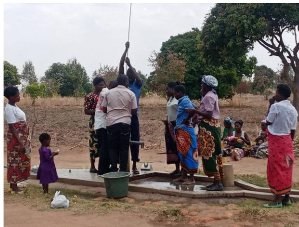
Borehole repair in Chadzerakuti village during the month
