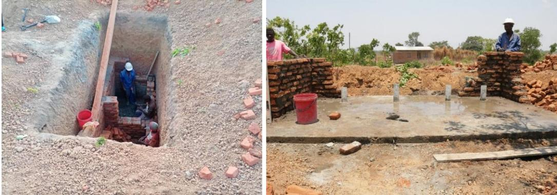
*Left - Construction of a sub-structure for the first block of pit latrines at Madzo Primary School, Right - Construction of the super-structure for the first latrine block at Madzo Primary School (Current status)*
