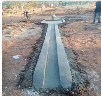
***Left** - Ngala Secondary school before civil works rehabilitation, **Right** - Ngala borehole after civil works rehabilitation before pump installation*
