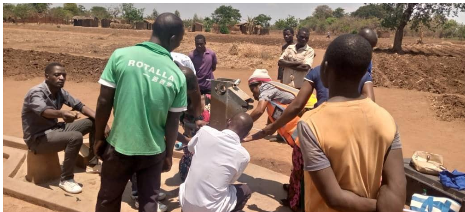
Borehole repair in Chiwoza village during the month
