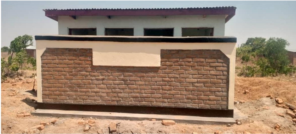
Pit-Latrines constructed at Madzo Primary School
