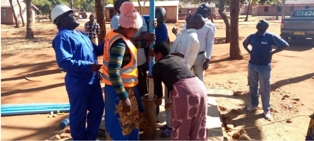
Team effort during pump repair at Chinguwi school during the month
