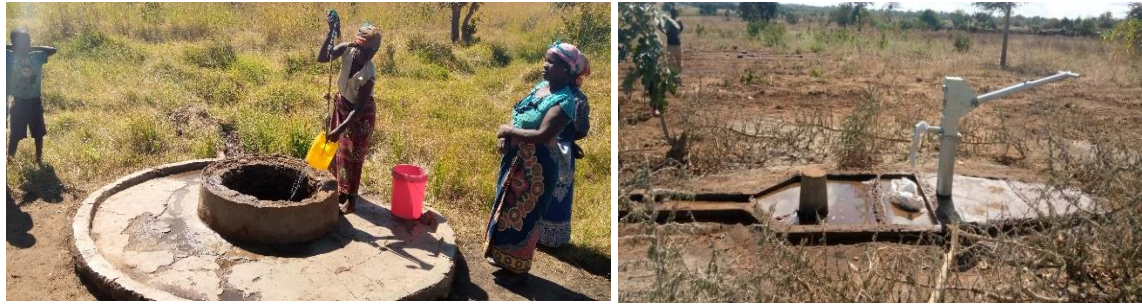
Left –Unprotected old water source in soko village, Right – New water source in Soko village during curing process before opening
