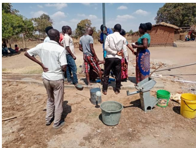
Team effort during pump repairs
