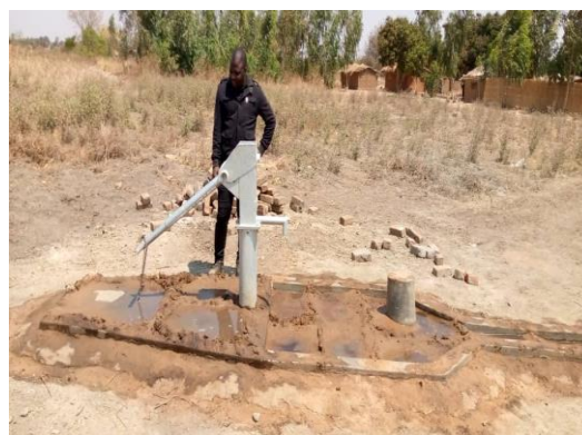
Left – Civil works at Kaunjika borehole, right – Civil works curing process at Chikumba before handover
