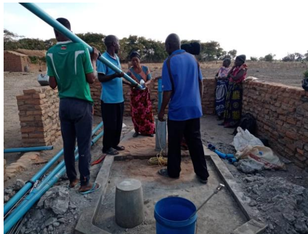
Team effort during borehole rehabilitation at Chiliphiza village during the month
