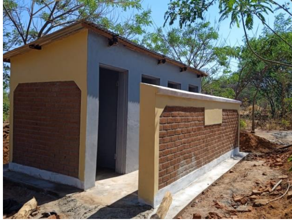
One of the newly constructed latrines blocks at Kapini school
