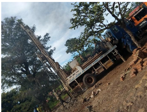
Drilling in progress
