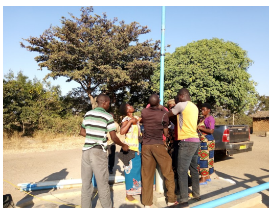
Images showing repairs in progress
