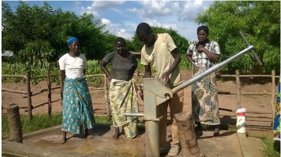
Figure 2: Community Member participating in borehole repairs
