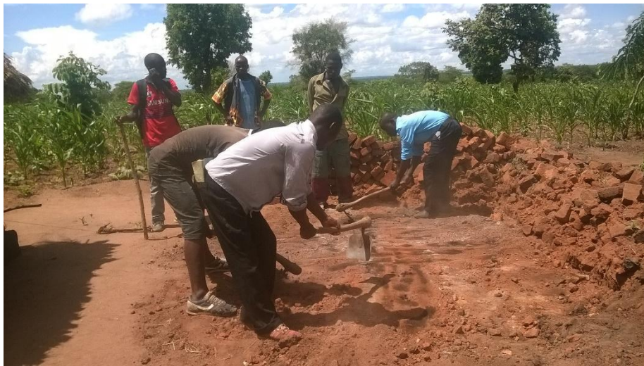
Figure 6: Trainees preparing where to dig a pit latrine
