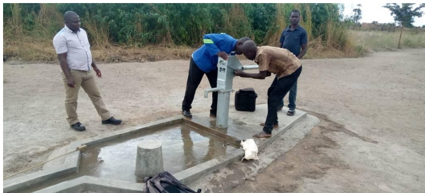
Pump repair session at borehole during the month
