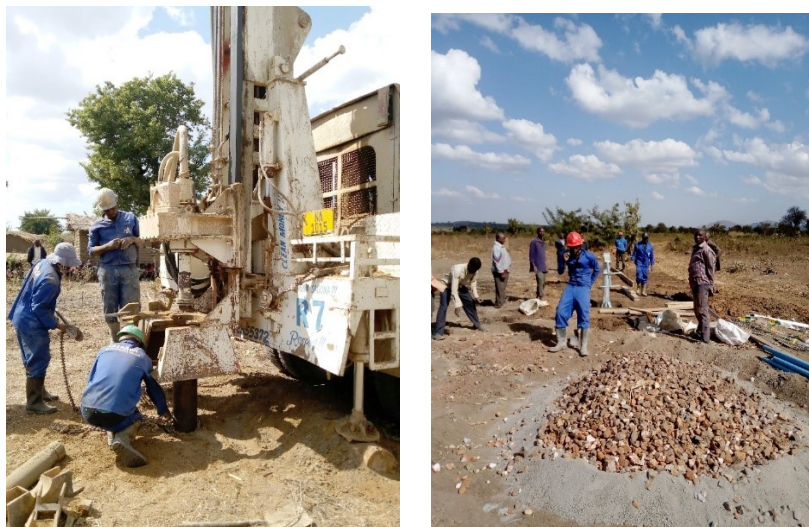
Images showing borehole drilling and construction works in progress
