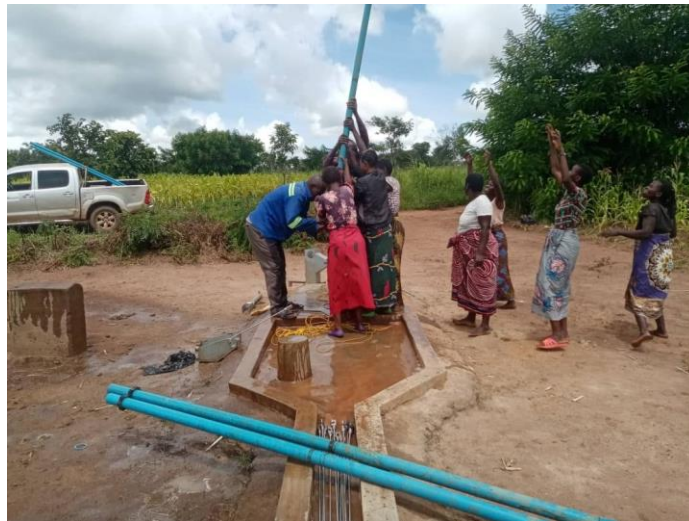
Pump repair session at Mimba water point during the month
