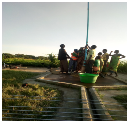
The community assisting during water well repairs
