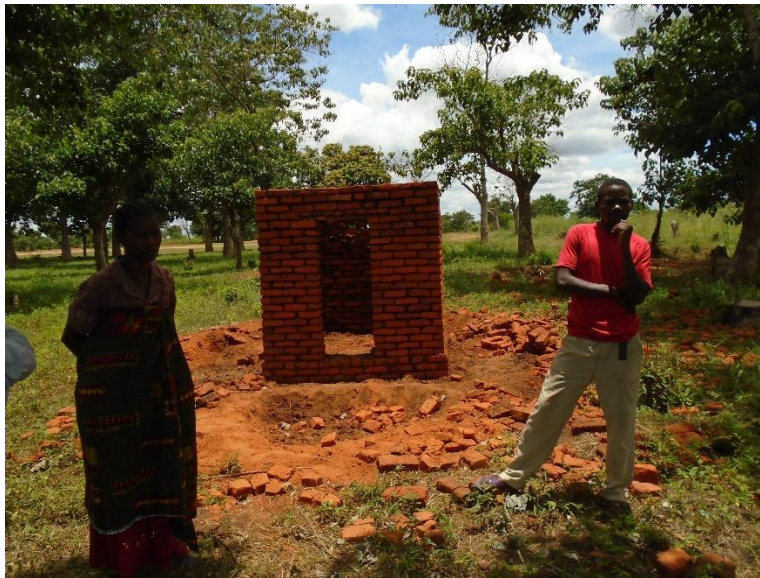
One of the constructed latrines before thatching
