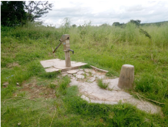
Image showing state of Kawiya borehole before the repair
