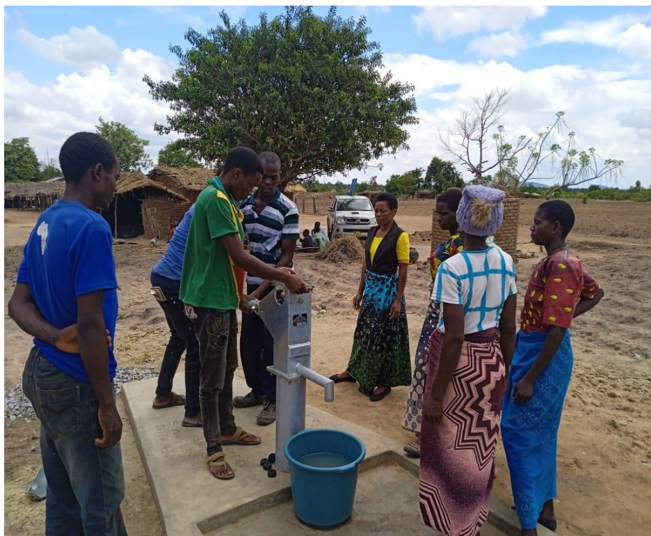
Pump repair session at Kasinja village during the month
