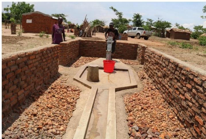
Newly drilled borehole at Katubede village, GVH Chimwendo
