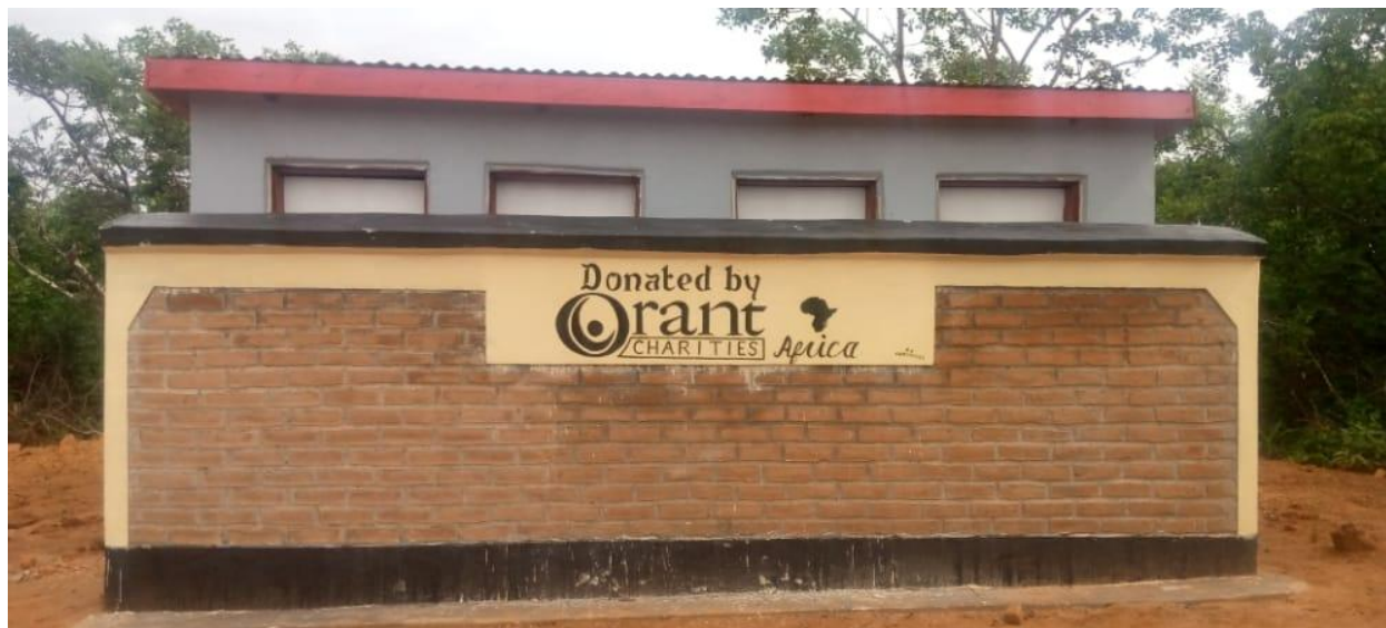
An improved pit latrine at Chilinkholi primary school
