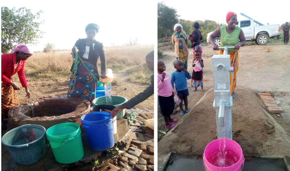
Image (left) showing the previous unprotected source and image (right) showing the newly constructed borehole.
