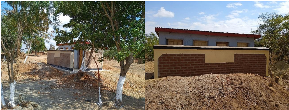
The new latrine blocks constructed by OCA at Nambola Primary school
