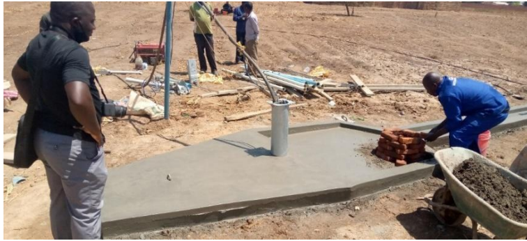
Kasese 2 Borehole during Pumping Test and Apron construction
