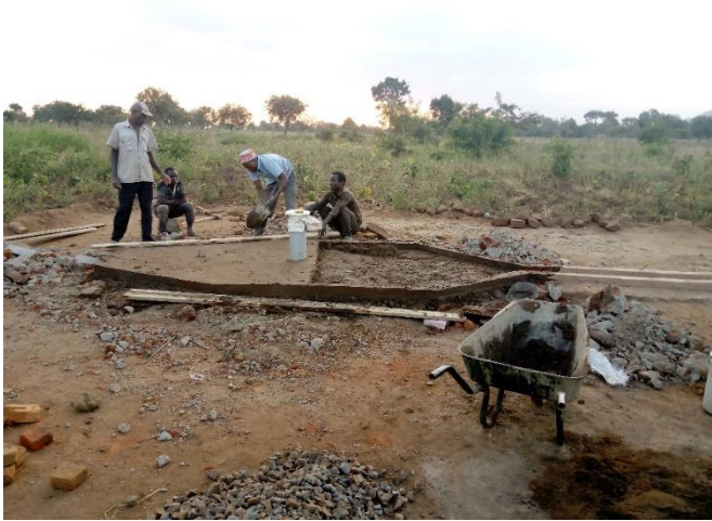
Part of the borehole rehabilitation works
